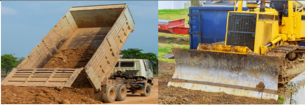
Fig. 2.18 Transport vehicles involved in the OFC installation
