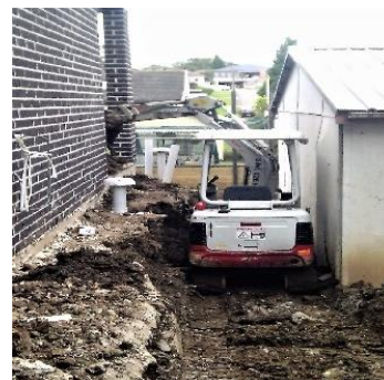
Fig. 2.8 Excavation in the open area Fig. 2.9 Excavation in narrow area using mini excavator
