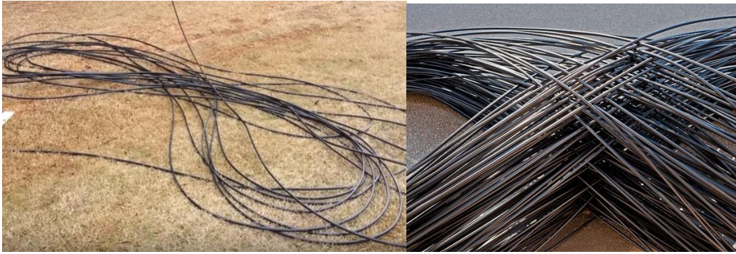
Fig.1.8 Right way to put the optical fibre cable on the floor
