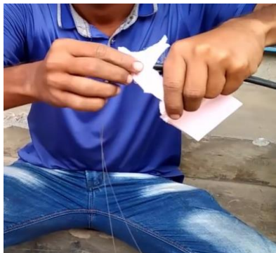
Fig. 5 Removal of the jelly around bunch of fibres with tissue paper
