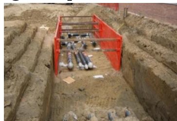
Fig.4 Bench in the trench
