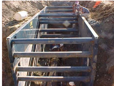
Fig. 2 Shielding of trench
