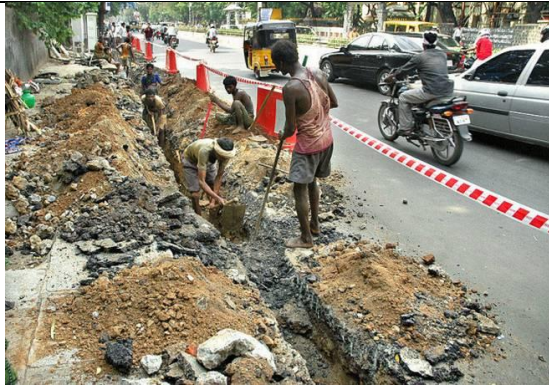
Fig.1.4 Men making the trench in urban area
