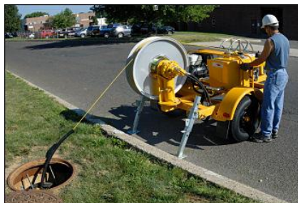
Fig. 1.10 Pulling machine pulling the optical fibre cable
