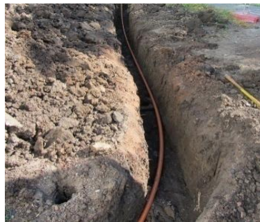
Fig. 1.6 Placing the cable in the trench
