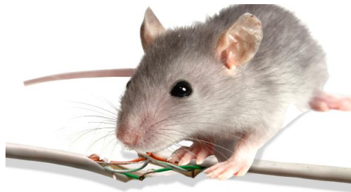
Fig. 2.4 Damage in the fibre cable due to rodent
