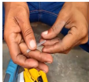
Fig. 5 Placing protection sleeve inside the fibre
