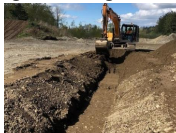
Fig. 3 Slope in the trench
