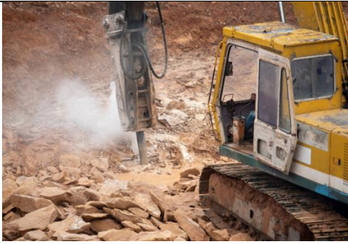
Fig. 2.15 (a) Excavation in rock
