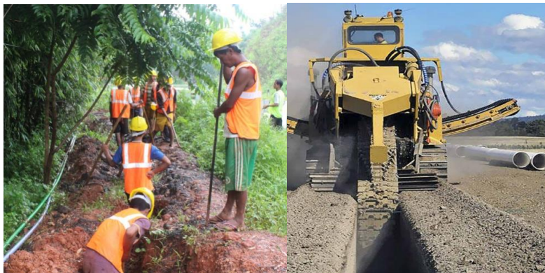
Fig.1.3 (a) Trenching using hand tools (b) Trenching using machinery
