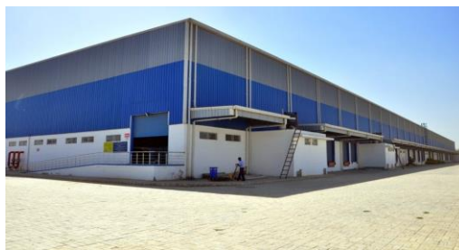
Fig. 2.19 Warehouse storage and ventilation
