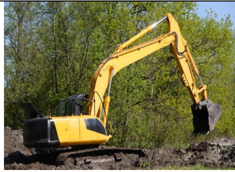
(b) Excavation in forest
