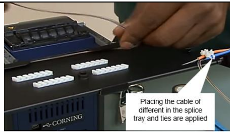
Fig. 2 Placing the cables of different colours in splice tray
