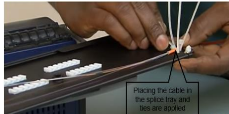
Fig. 3 Placing the cable in splice tray and ties are applied
