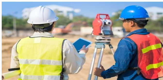
Fig. 2.1 Team performing site visit
