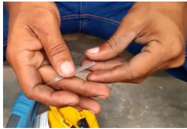
Fig. 6 Placing protection sleeve inside the fibre
